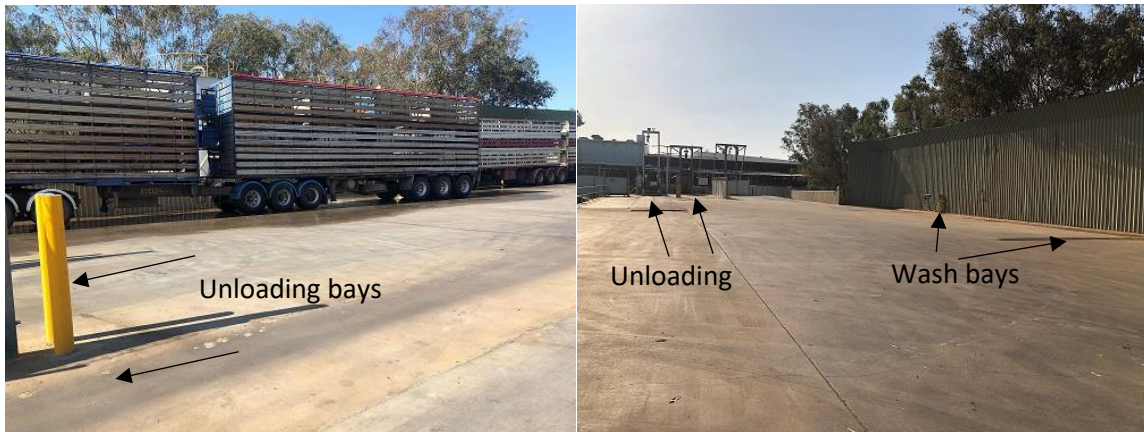
Figure 1: Current truck wash facilities at Linley Valley Pork
