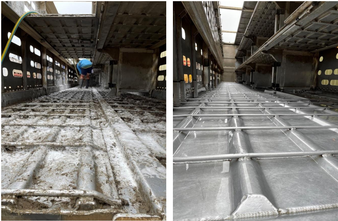
Figure 4: Applying foam detergent (left) and after hosing (right).
