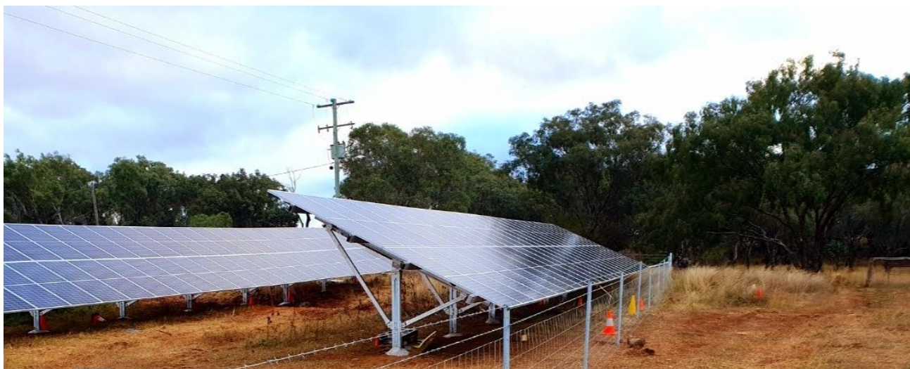
Figure 30. Installation of a 39.36 kW ground mounted solar system with a 2 x 15 kW inverters. Source: Queensland Farmers' Federation, n.d.
